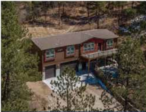
9140 FRANK ROAD | LARKSPUR | UNDER CONTRACT! | OFFERED AT $775,000
