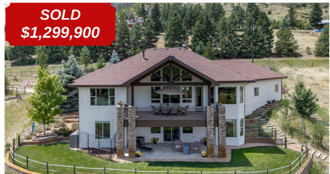
2359 Valley Park Drive - Valley Park
