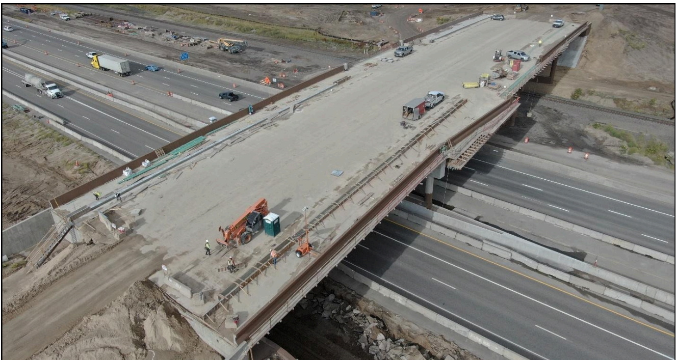
Crystal Valley Parkway bridge over I-25 in September 2025
